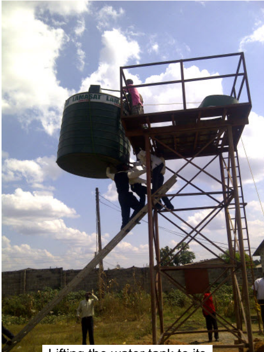
Lifting the water tank to its new position
